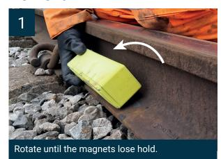
The device must be placed on the smooth part of the rail web.
