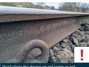
Don't place the device on rail joints or rail branding.
