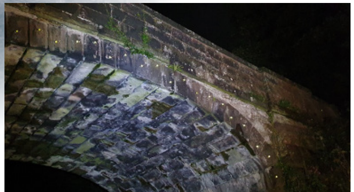
Monitoring targets installed on arch of Rosegyhll Bridge
