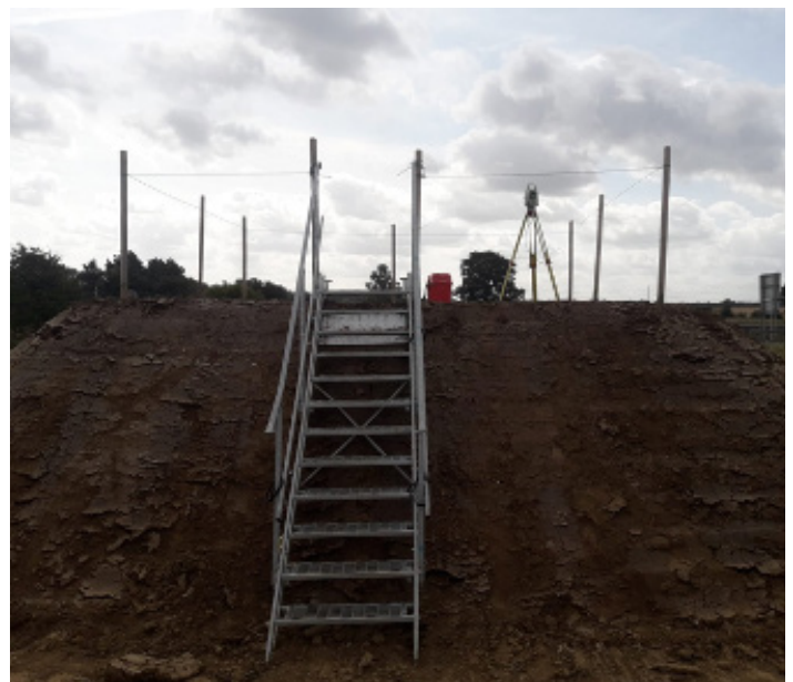
Monitoring platform – to provide sufficient line of sight
