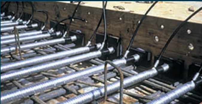
TYPICAL THREADBAR® TENDON INSTALLATION, AERATION/EQUALIZATION BASIN MCINTOSH, AL
