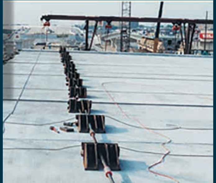
TEMPORARY THREADBARS FOR PRECAST SEGMENTAL CONSTRUCTION
