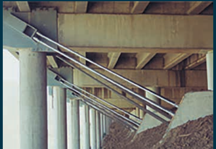
BRIDGE REPAIR THREADBAR® STAYS ROUTE 580 ALTAMONT PASS, CALIFORNIA
