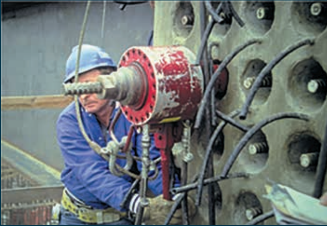
THREADBAR® STRESSING OPERATION MOPAC FREEWAY/US 183 INTERCHANGE AUSTIN, TX.
