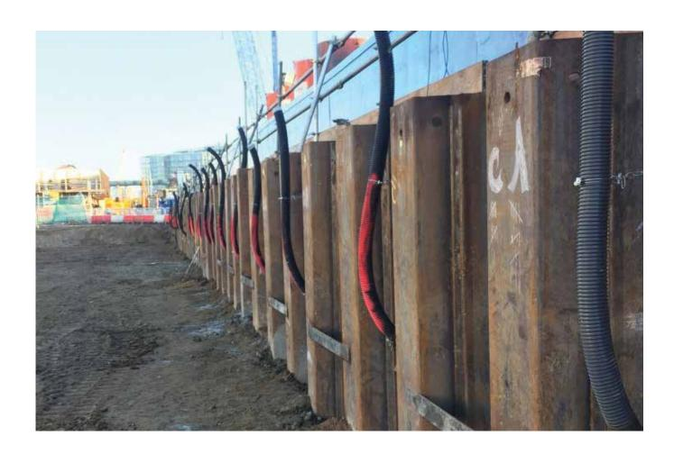
When temporary anchors are installed into ground that has potential for future development, an alternative solution to the removable anchor system is the cuttable anchor. Glass Fiber Reinforced Polymer bar has been used for passive systems such as rock bolts and soil nails for some time; however, as a material which is easily cut, it can provide specific qualities desirable temporary pre-stressed systems too.
