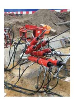
BS8081 defines permanent anchors as installations with lifespans in excess of 2 years. In order to achieve this status, sufficient corrosion protection needs to be provided. To ensure durability throughout the working life of each anchor, double corrosion protection needs to be provided. Double corrosion protection (DCP) is defined in BS8081 and consists of factory pre-grouted encapsulation of the bar within a corrugated plastic sheath.
