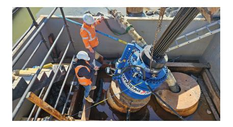
DYWIDAG provided a comprehensive solution through the design, manufacturing, and installation of advanced multistrand anchors. These 61-strand anchors, reaching lengths of up to 40 meters, were installed within large steel foundation piles, which were driven at an angle into the seabed rock. The bond length of the anchors extended through these piles into the deeper bed rock, securing a strong connection between the subsea rock and the market's foundation.
