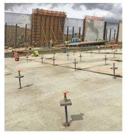
DYWIDAG was part of the emergency recovery team. DYWIDAG produced and supplied 7096 epoxy coated DYWIDAG THREADBAR® 36mm anchors in varying lengths 4.6m-7.6m long. DYWIDAG anchors were also used for the anchoring of the concrete slab
