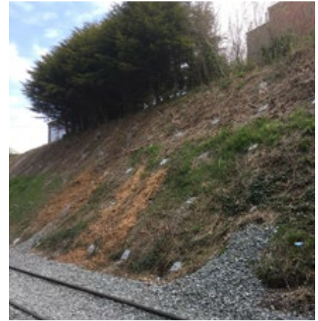
Slope stabilisation at Phoenix Park, Dublin
