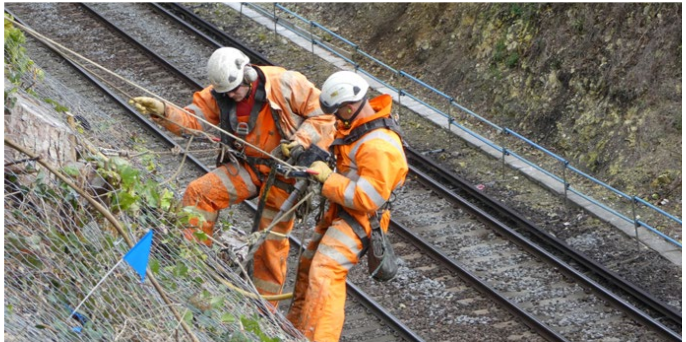
Hand drilling through DELTAX® at Hove
