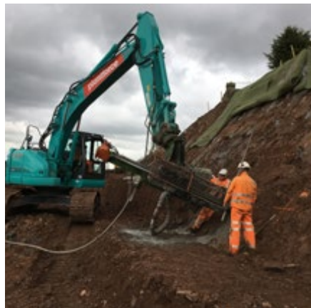
Excavator mounted rig at HoTV A465
