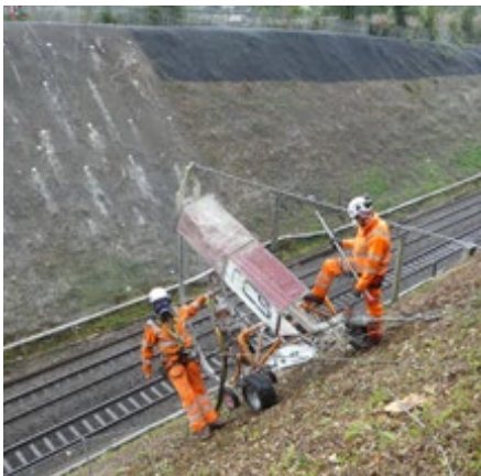
A Frame drilling at Watford Cutting
