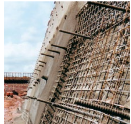
Grouted soil nails on shotcrete face
