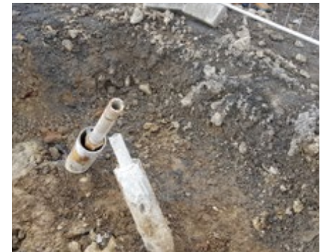
Raking T76 Micro Piles
