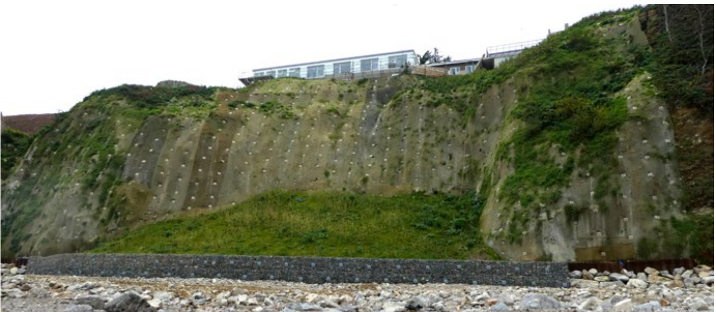
GREENAX® enables vegetation to establish on steep slopes, providing further reinforcement to the cliff face.
