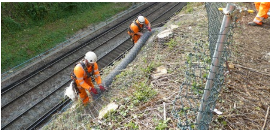
DELTAX® mesh being laid over tree stumps in Hove
