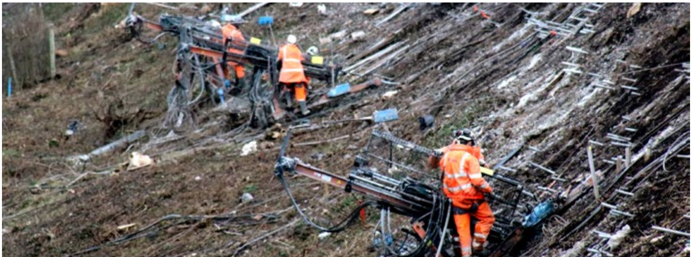
Soil Nailing using DYWI® Drill Hollow Bar at Filton Banks, Bristol
