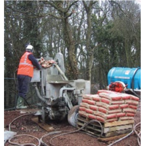
Typical grout plant set-up
