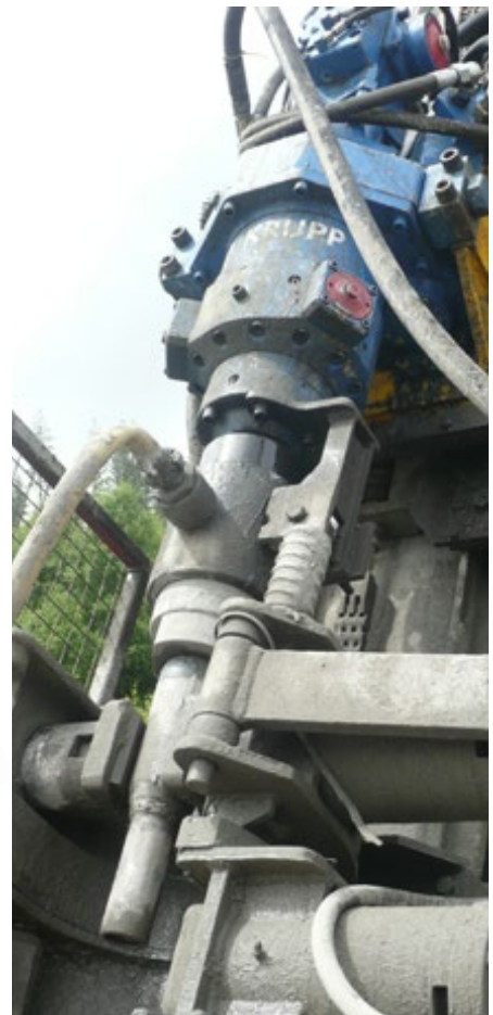
Drill head with simultaneous drill & grout feed
