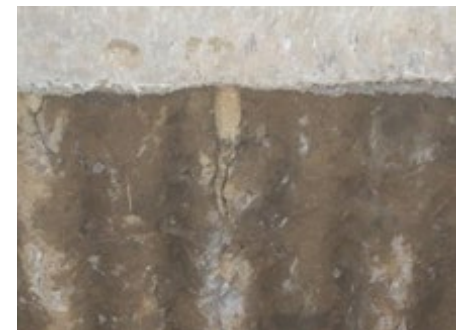
T76 Micro Piles forming a contiguous wall
