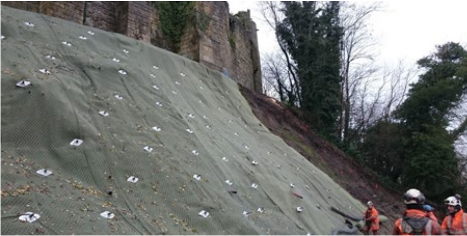
Soil Nailing using DYWI® Drill Hollow Bar, DYWI® Mat Green & TECCO® G45/2 Cockermouth
