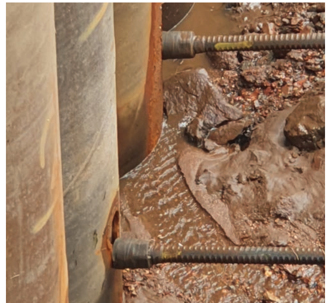
Owner: AV Dawson Ports General contractor: TMS Maritime Ltd Products supplied: 63.5mm GEWI® Tie bar and gusseted plates
