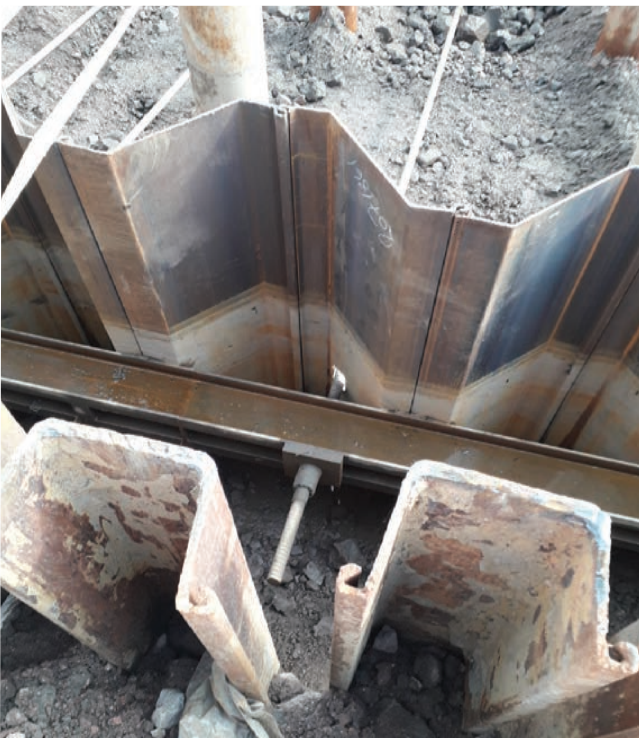
Owner: AV Dawson Ports General contractor: TMS Maritime Ltd Products supplied: 63.5mm GEWI® Tie bar and gusseted plates
