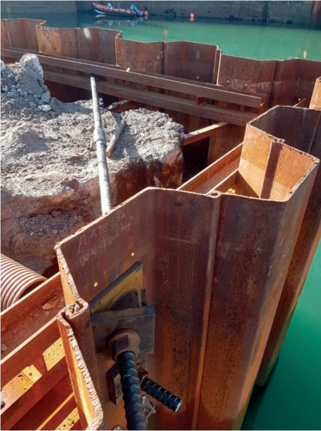
Owner: Aberdeenshire Council General contractor: TMS Maritime Ltd Products supplied: 50mm GEWI® Tie bar
