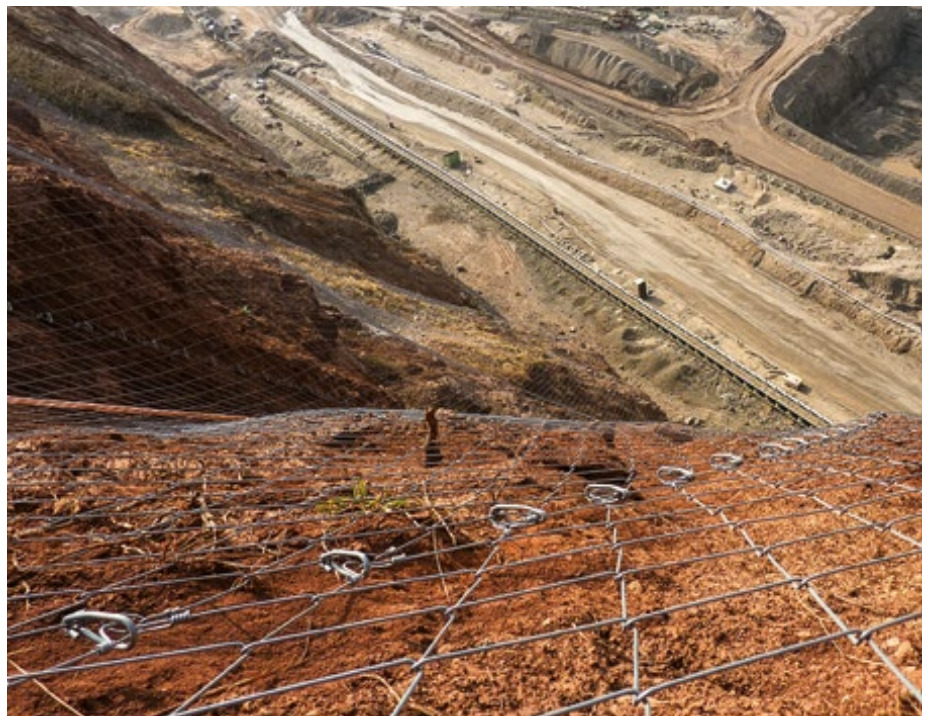
T3 clips - used to connect adjacent mesh panels together.
