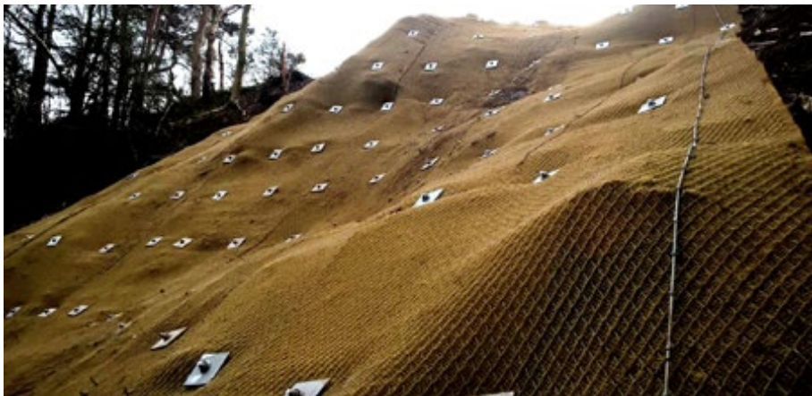
TECCO® Green - Installation at Castle Eden Dene
