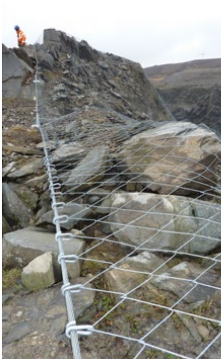
T2 clips - used to connect the mesh with the boundary wire rope
