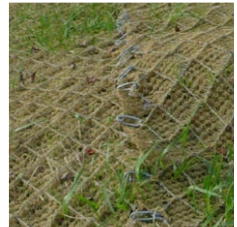
T3 clips - used to connect adjacent mesh panels together.
