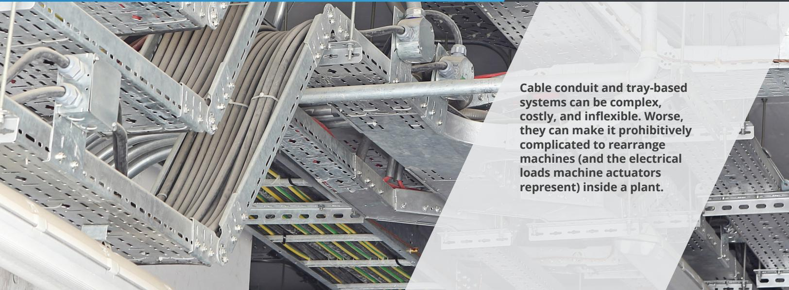
Cable conduit and tray-based systems can be complex, costly, and inflexible. Worse, they can make it prohibitively complicated to rearrange machines (and the electrical loads machine actuators represent) inside a plant.
