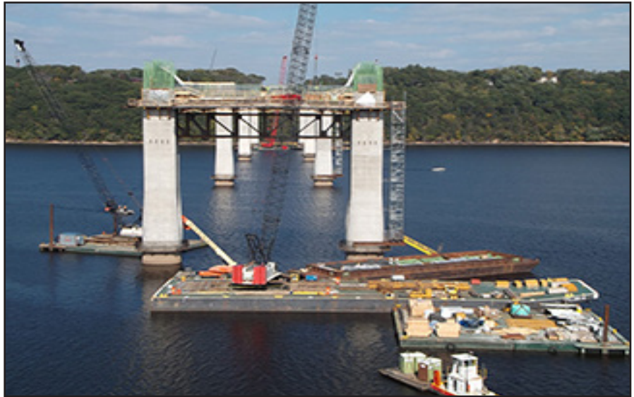
Construction of bridge piers 9-12, August 2014 Photo courtesy MnDOT
