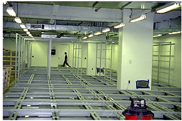
Compactor Carriages Installed in New Vault
