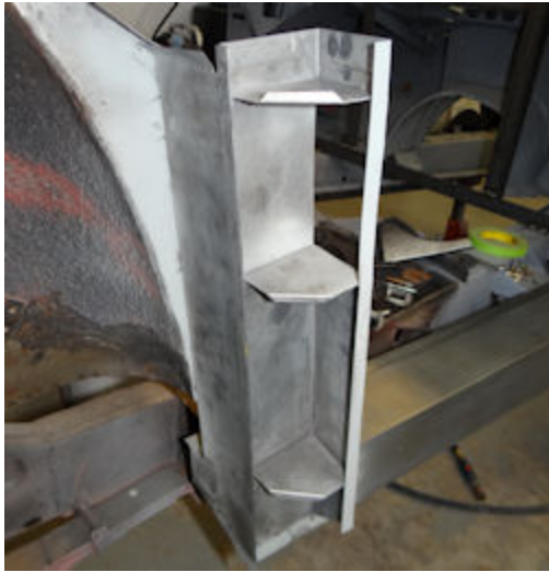
Inner B pillar structure now welded in position
