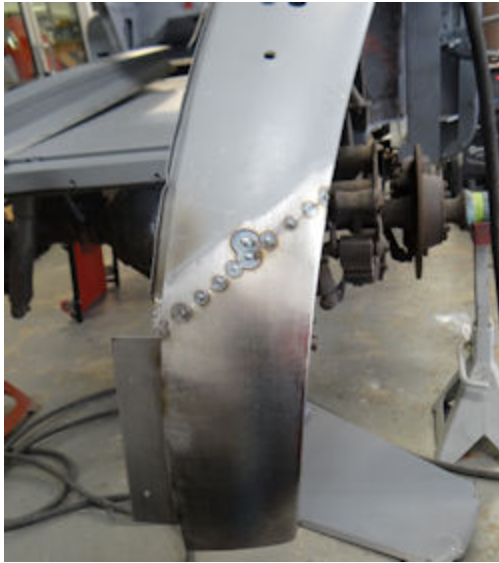
New panel is first tack welded in place
