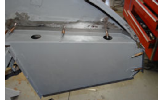
Slowly but surely, the affected area is reconstructed
