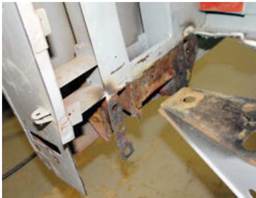
Significant rust inside A pillar
