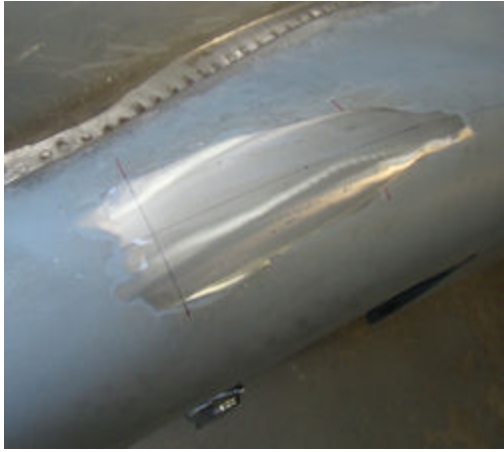
With TIG beads cleaned up, repair is virtually invisible
