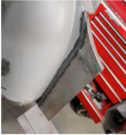
Seam is then TIG welded
