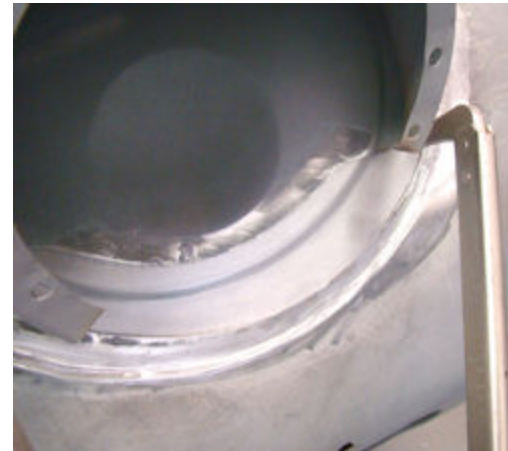
Repair panel fabricated and clamped in place
