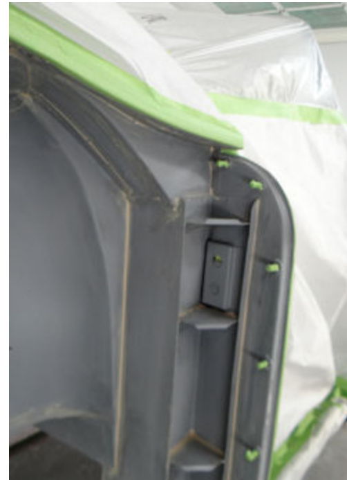
Seam sealer applied to all seams and joints in B pillars, firewall and inner wheel arches
