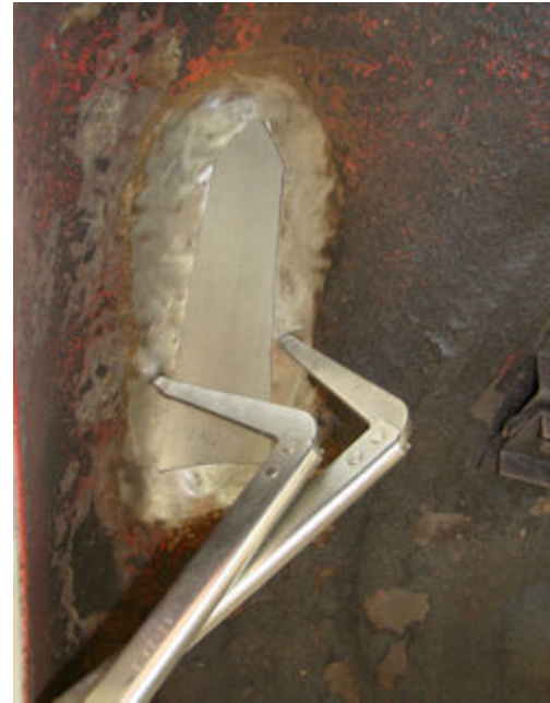
Panel will be trimmed to fit the hole exactly
