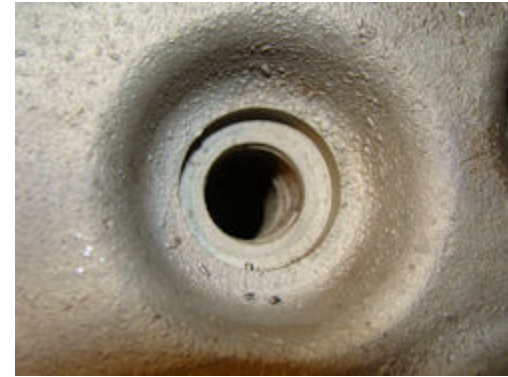
Stripped out spark plug holes will be repaired
