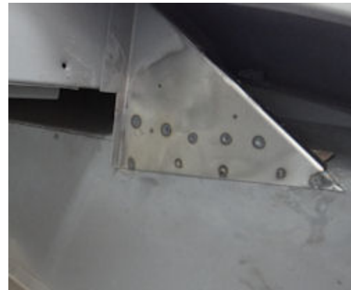
Rust cut out, new panel fabricated and welded in place
