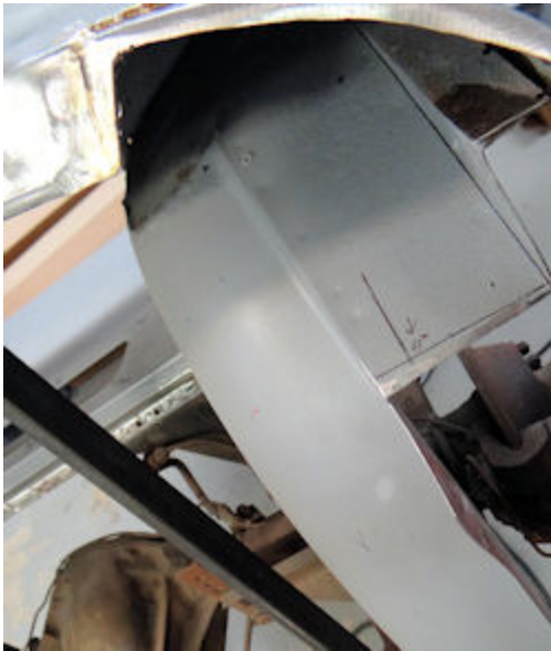
With corroded metal cut away, there isn't much left
