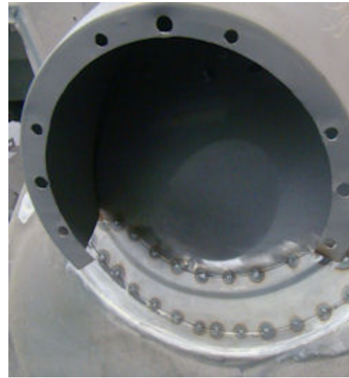
Tack welded in position
