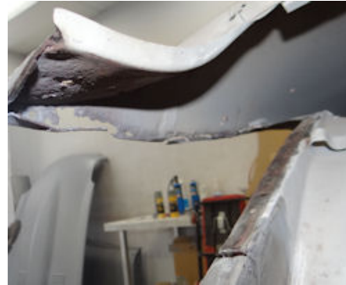
Last photo in this sequence shows this area reconstructed
