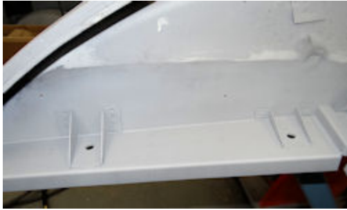
Side panels fabricated and welded in place
