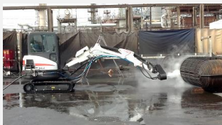
PSC uses an automated hydroblaster to clean a heat exchanger
