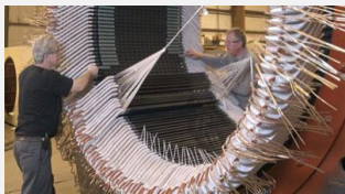
IPS repairs a large electric motor for a petrochemical facility
