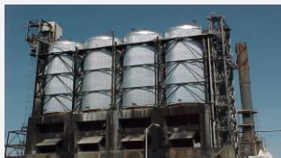
Ardent completes new substation tie-in and coker turnarounds
