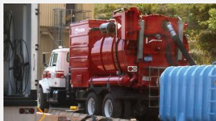
HydroChem uses a specialized vacuum setup for coating removal
