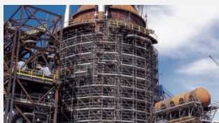
Brand uses scaffolding for refinery tank maintenance
