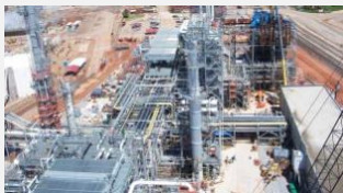
Zachry/JVIC conducts a turnaround at the Phillips 66 refinery in Borger, TX
