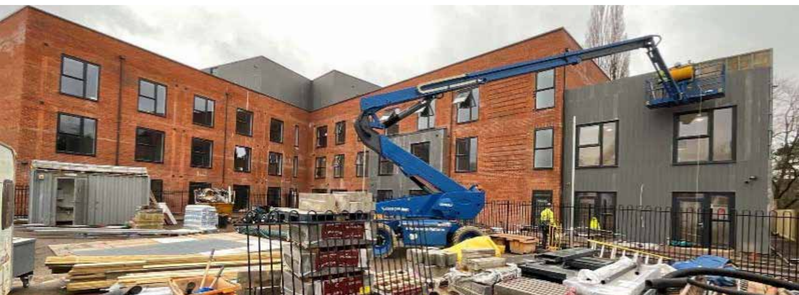
Grand designs – the new Shenstone Court development is really taking shape!
