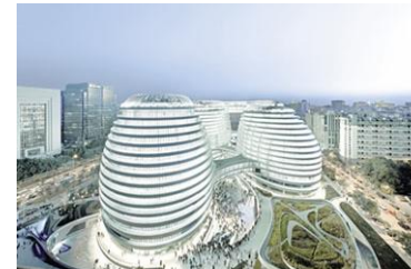
Galaxy Soho Office Building, Beijing (China)
