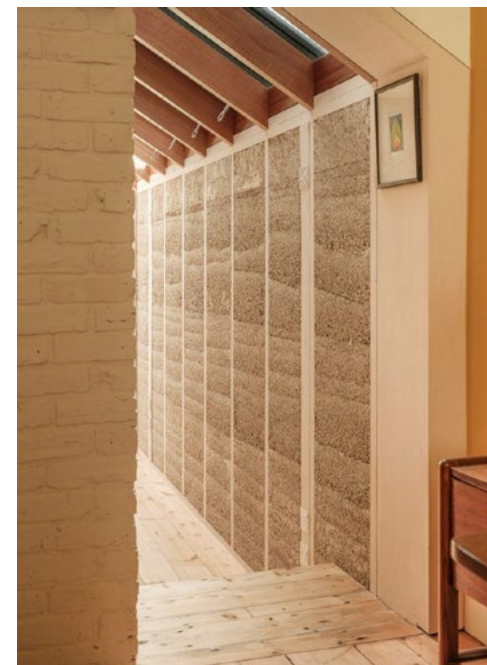
House Made by Many Hands by Cairn, East London. Hemplime was poured in place between framing and left exposed, with art hung on studs. Ready-made panels of hemplime could be painted with mineral paint, with art mounted to framing.
