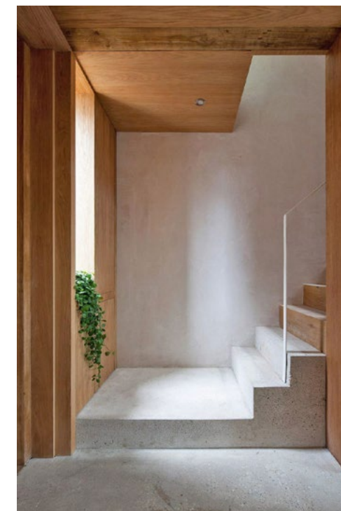
Hempcrete Mewshouse by Cathie Curran studio, East London. Hemplime block construction with lime plaster.
