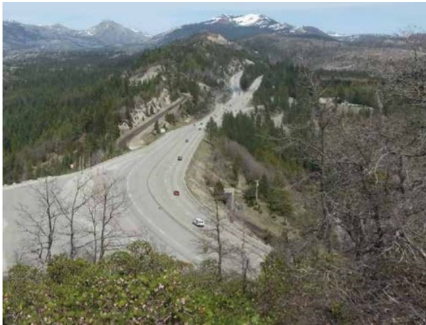
Two views of Emigrant Gap Ridge between Bear Valley and the North Fork of the American River at an elevation of 5300 to 5500 feet. The original railroad grade is shown above in 1867, while the lower image was taken in 2015, showing Interstate 80 sharing the narrow drainage divide, with the rail line crossing beneath (upper image is from the Alfred Hart Collection-Stanford Archives; lower image from Donner Summit Historical Society).
