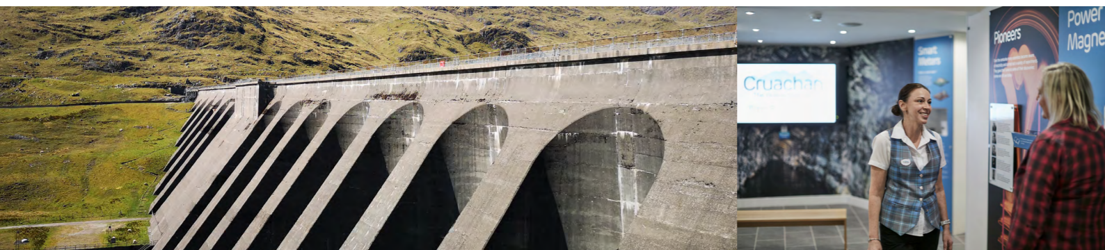
Photo: Cruachan Dam, Cruachan Hydro Power Station
