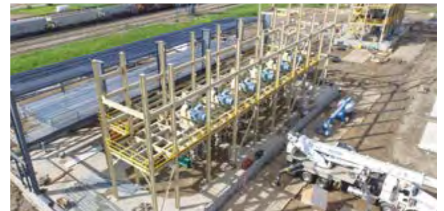
Photo: High Level plant in early construction
