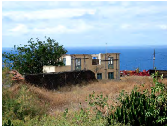
View of the Yellow House—looking northeast
