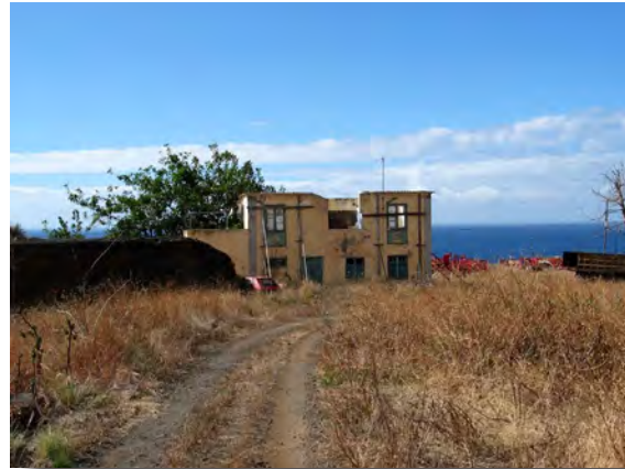
Approaching the house from the east
