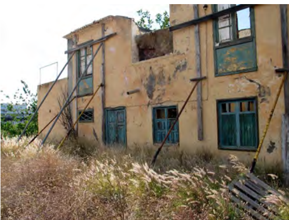
Southern facade, showing braces on the walls
