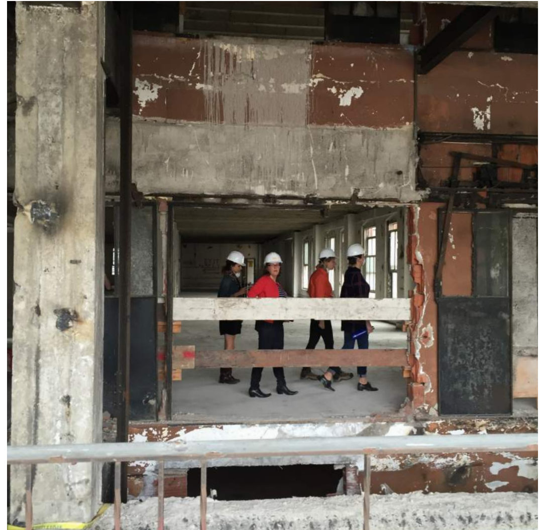
Broadway Trade, Under Construction
