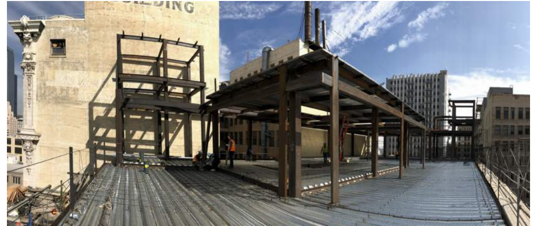
Desmond's, Rooftop Addition Framing
