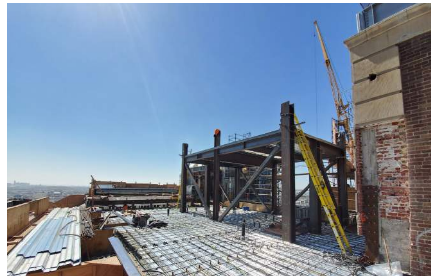
Proper Hotel DTLA, Rooftop Addition Framing
