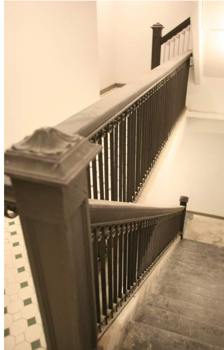
Broadway Lofts, Historic Stair Guardrail
