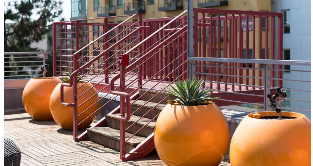
Residential Amenity Deck, New Stairs and Landing at Fire Escape
