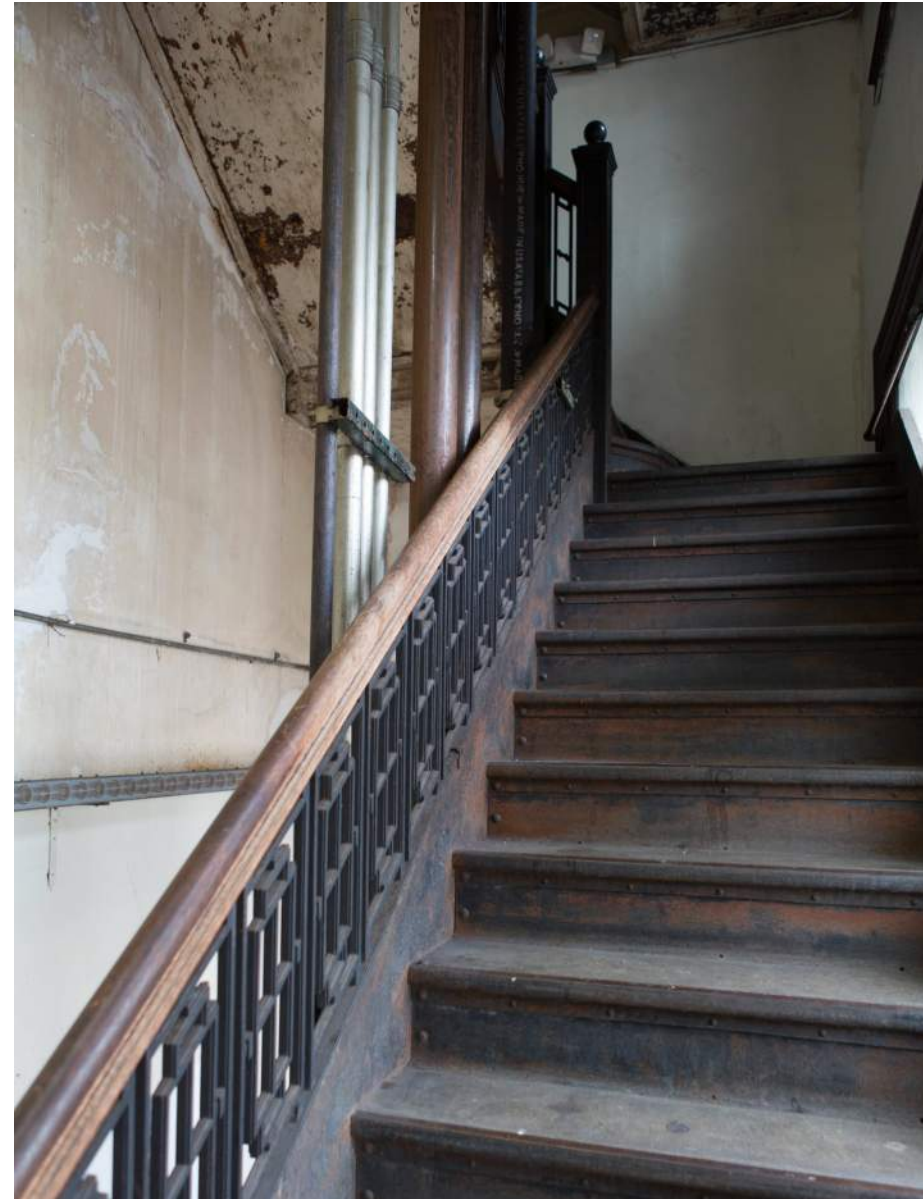
Broadway Trade, Existing Exit Stair
