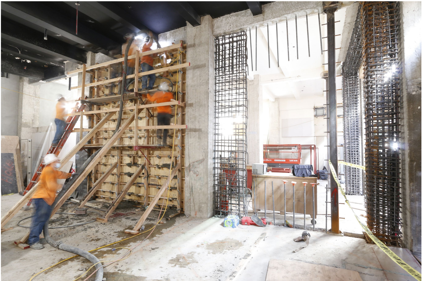
Lane Building © Reaume Richardson
