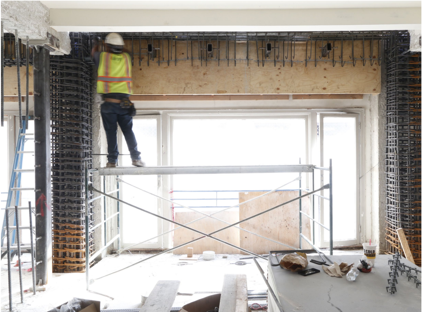
Lane Building © Reaume Richardson
