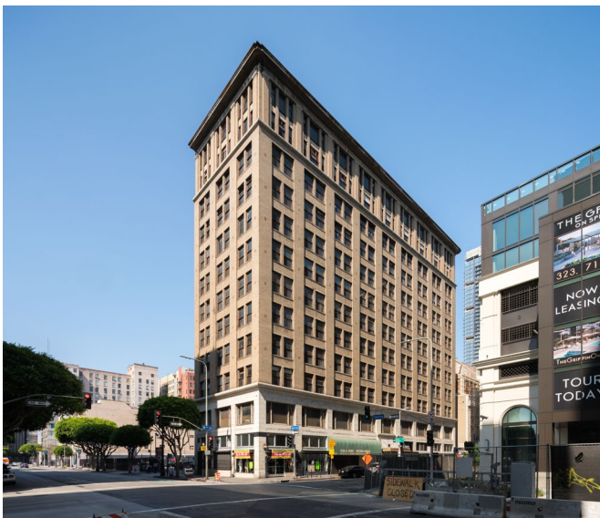
The Lane Building, adaptive reuse from office to housing, under construction. © Hunter Kerhart
