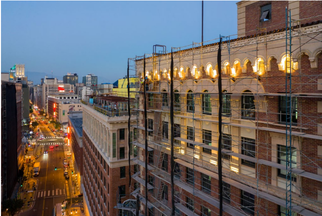
Proper Hotel looking North on Broadway © Hunter Kerhart
