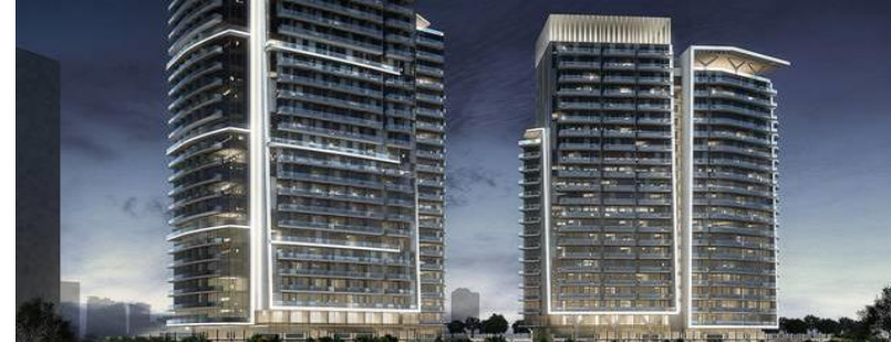
Mid rise Apartments
