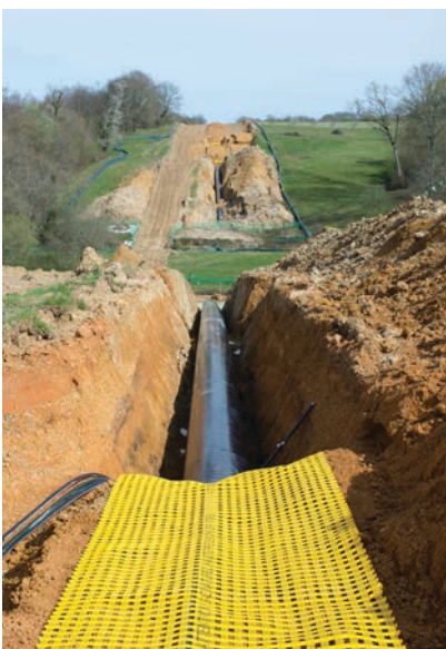
Gas pipeline before being lowered into the trench
