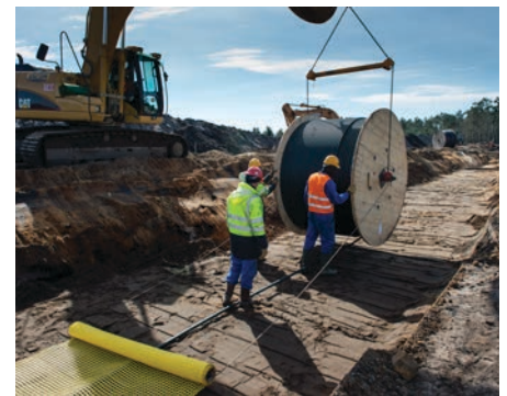
Fibre optics being laid before pipework is lowered in
