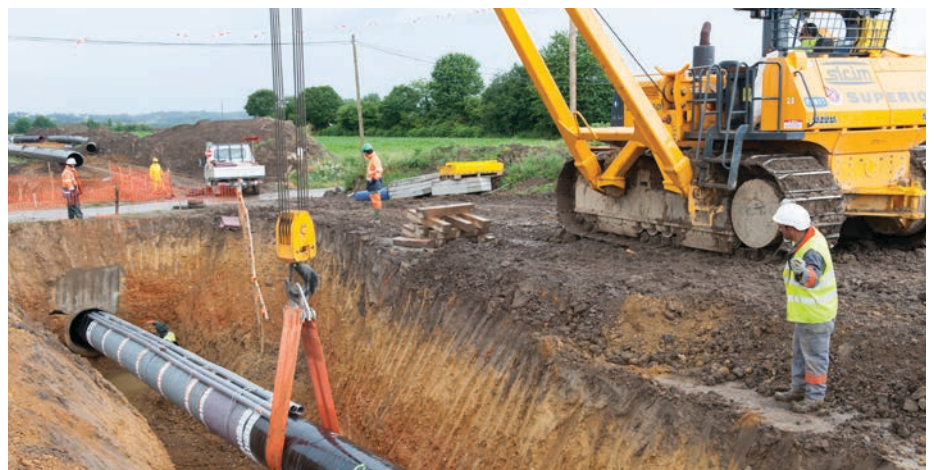
A pipeline being inserted into its duct under a road
