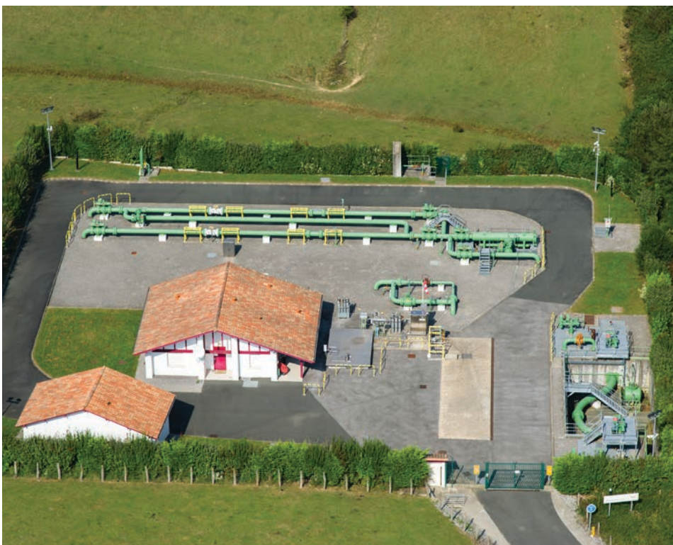
Urrugne switching station
