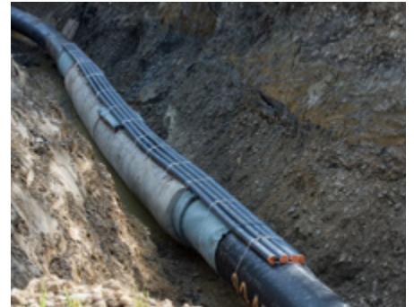
Optical fibres installed in their ducts alongside a pipeline.
