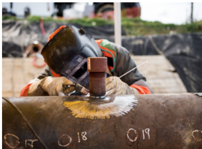
Repairing a gas pipe.
