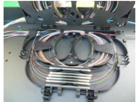
Optical fibres drawer at the Saint-Justin station.
