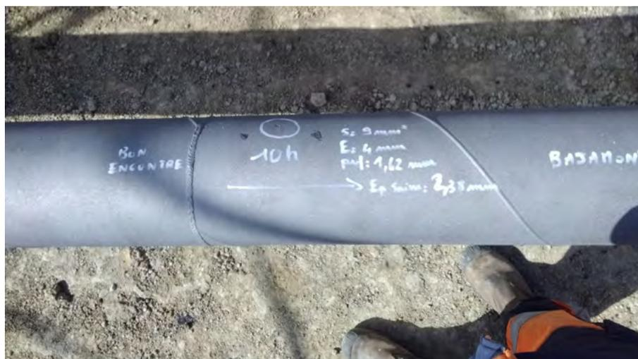
Pipeline with indication of defects.
