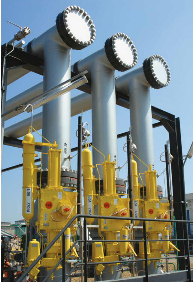
Equipping the Lussagnet storage platforms.
