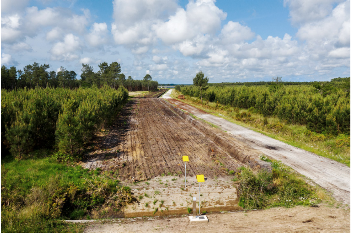
Bolstering the Rion-des-Landes gas pipeline.
