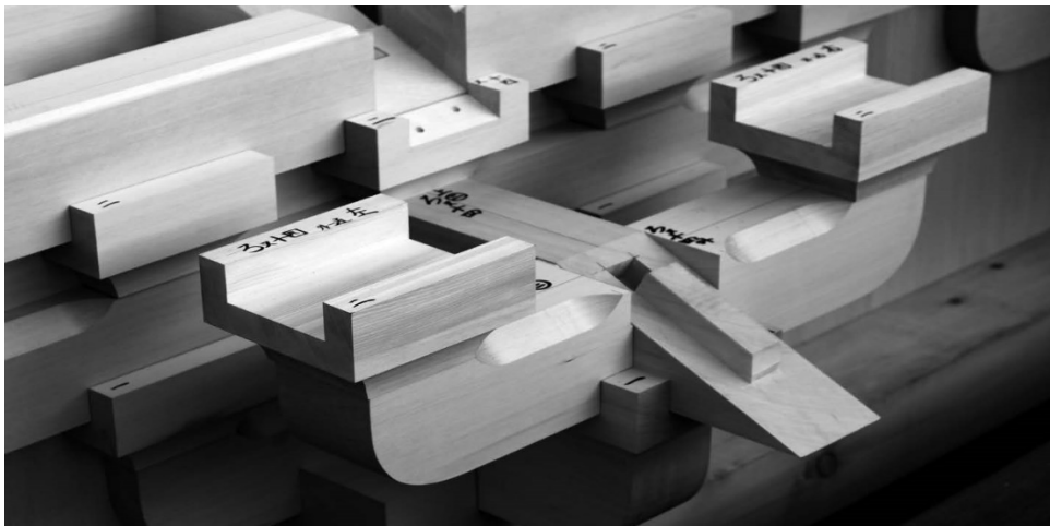
Assembly of a bracket complex. Courtesy of Takenaka Carpentry Tools Museum
